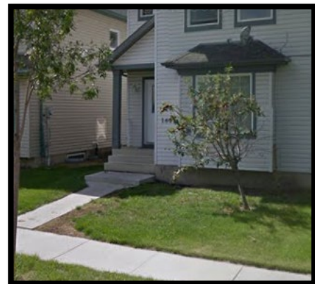
Sod dead, tree leaning over and needs to be staked
